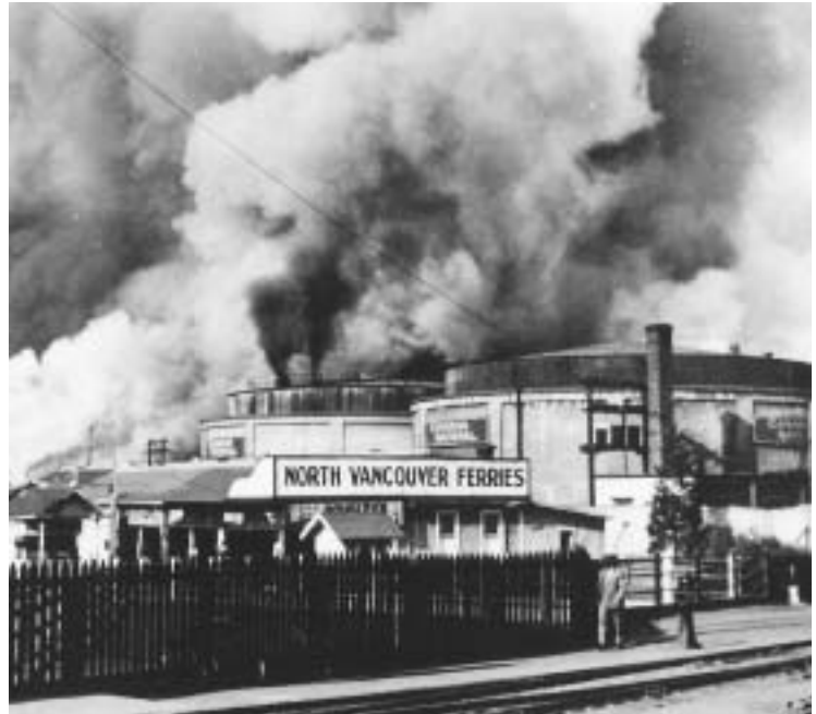
Canadian National Dock general alarm fire. Photo: VFD Archives
