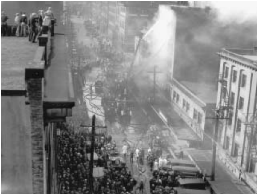
The Slade fire looking west to Cordova Street. Photo: CVA 99-2450
