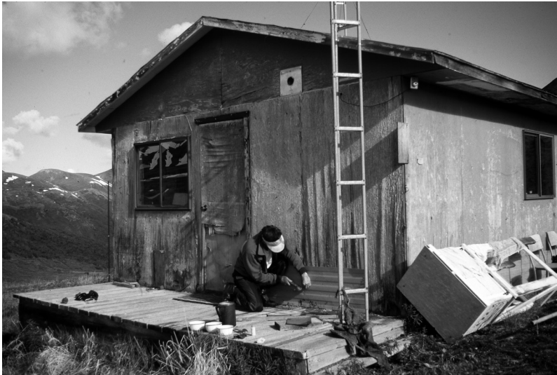
John repairing the Potato Hill cabin.
