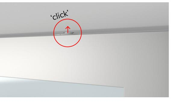
Now all 4 positioning caps are in place, further adjustments can be made safely.
