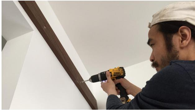
Use provided  $5/16'' \times 4''$  lag bolts and spacers to fasten the track to the wood block. Note, the flanges on the spacers are to face the wood block. Check for level and adjust if necessary.
