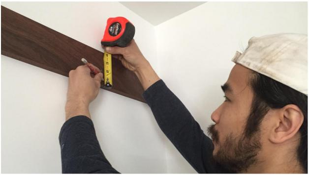
Lay the track on the wood block and mark the drilled holes onto the wood block. Make sure the track is leveled.
