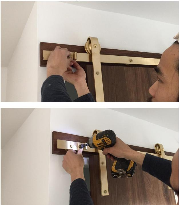
NOTE: Usually, stoppers can be installed on the last hole on both ends of the track so that new holes do not need to be drilled
