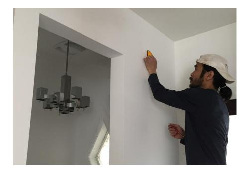
2. Install wood block (This step can be omitted if barn door track is installed directly on the wall) Mark on the wall the location of the wood block. The wood block is installed at 0.5" higher than the height of the door. Example: if the door is 80" high, the height from the floor to the bottom of the wood block is 80.5"
