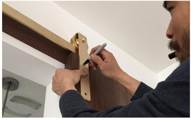
Use 3/16" drill bit to drill marked holes.
