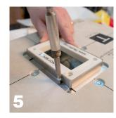
Fasten the tile dam using the four mud dam screws. Be sure to use a low torque setting so that the tile dam is not distorted. Also, if longer screws are needed, any standard #6 pan head screw can be used.
