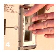
Insert the tile dam into the opening. Make sure that the plastic box fixture is pushed all the way in to ensure that the tile dam is centered on the enclosure.
