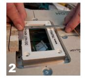
Lay in tile dam with plastic fixture and determine amount of shims needed. Tile dam is best fitted slightly lower than the tile height. Remember to compensate for mud behind tile.
