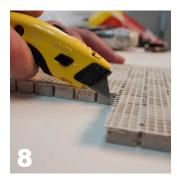
Cut tile - grinder or tile saw may be needed to cut individual tiles.
