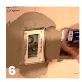
Apply mud using standard industry practices being sure to fill the area around the tile dam before applying a notch trial finish.
