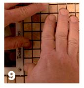
Set tile - being mindful of keeping an equal grout line around device.
