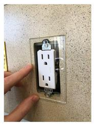
White metal backplate safely covers electrical box, if used without backplate you would see into wall.
