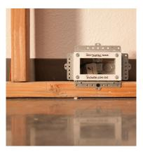
Remove the enclosure from the panel and fasten it directly to the framing in its approximate location. Leave it in this location until all wiring has be terminated in the opening. Be sure to terminate wiring through the rear plate only unless a deep box accessory is being used.
