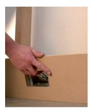
Attach the enclosure to the baseboard - per TRUFIG Install Guide procedures for Solid Surface (wood) - and reattach the back plate to the enclosure. The baseboard is now ready to secure to the wall.
