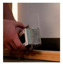
When the opening in the baseboard has been routed - use either the TRUFIG router templates, or a CNC machine to cut a precise fascia opening. See the TRUFIG Install Guide for more details on a solid surface install - remove the back plate from the enclosure and unscrew the enclosure from the framing.
