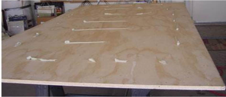
Spread Panel adhesive on plywood to adhere foam board insulation
