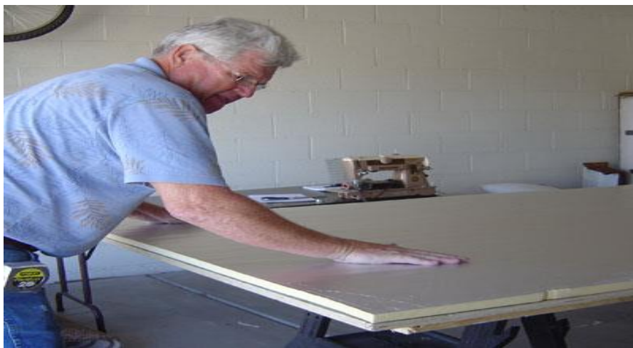
Applying the foam board insulation
