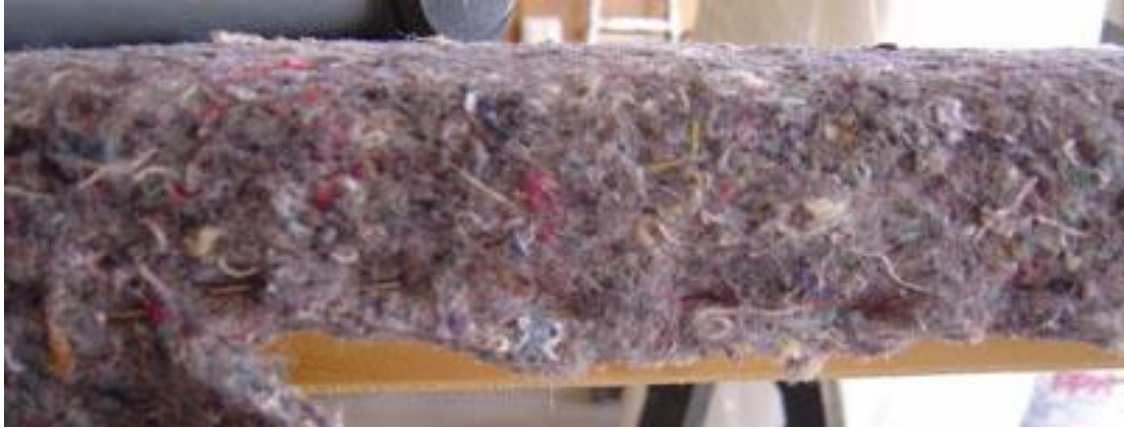
Apply a layer of auto thermal carpet pad insulation
