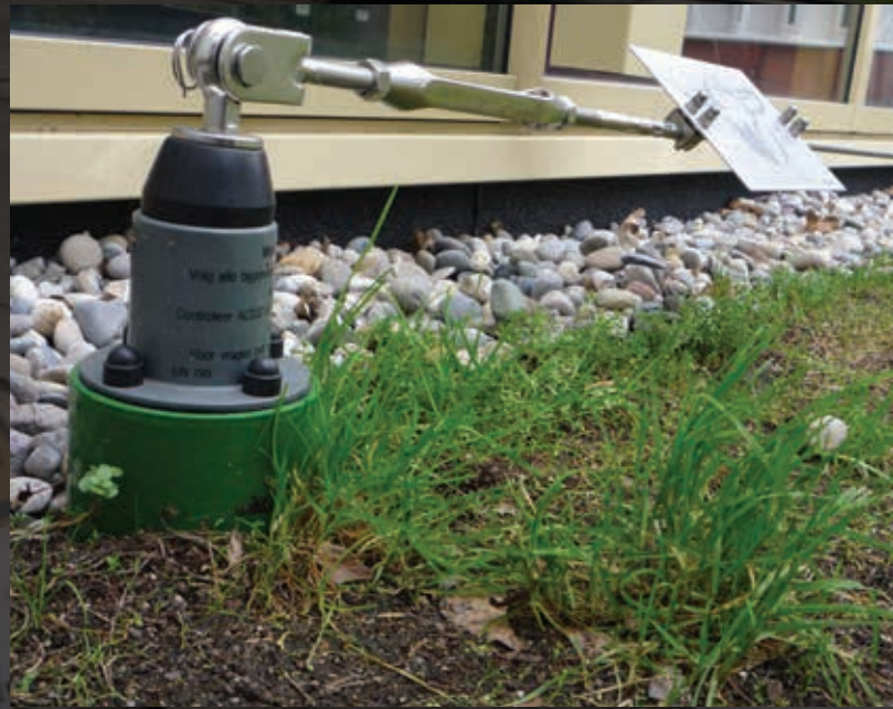
Green Roof Riser Post
