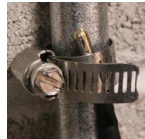
(4) Use an adjustable galvanized hose clamp.
