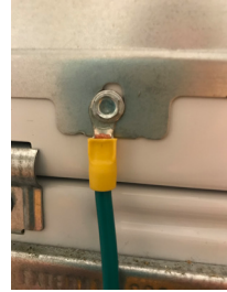
(1) Ring terminal installed on dryer.
