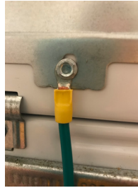
(1) Ring terminal installed on dryer.
