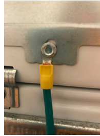
(1) Ring terminal installed on dryer.
