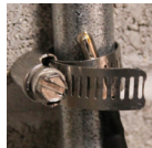
(4) Ground Pin Clamped Using Hose Clamp.
