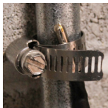
(4) Ground Pin Clamped Using Hose Clamp.
