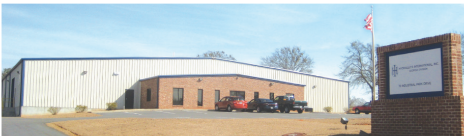
AIRCRAFT COMPONENTS AND GSE MRO FACILITY
