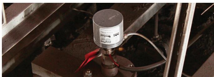
The Oxyfire™ In-Situ Zirconia Oxygen Sensor is designed to measure excess oxygen in combustion processes
