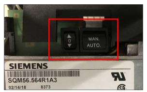
Set the switch to "MAN" and use the up/down arrows to move the actuator.
