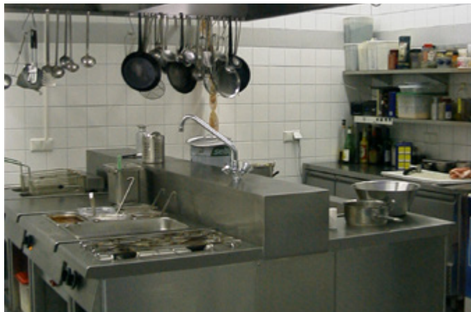
Filter monitoring in kitchens
