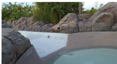
The Foam Armor™ system typically consists of an easy to use Base Coat 3150 applied between 100-250 mils and then top-coated with 2205, an aliphatic, abrasion resistant, color stable polyurethane elastomer. The combined system provides a tough impact and puncture resistant monolithic membrane that is slick and resist mold and calcium build up. The base-coat can be brushed applied and the topcoat is recommended to be sprayed. More info can be found on our website: www.waterparktech.com
