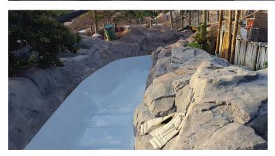
major water park had a concrete slide lined with EVA foam that was having topcoat degradation. Running the park 7 days a week with high UV and millions of gallons of water pouring over the surface, it had seen better days. The Park had been using the Creative Polymers Foam Armor™ and Slide Armor™ systems on other park maintenance with great success, so it was determined that the Foam Armor™ could do well here too. The system had passed a 5 year test study for performance with excellent results.
