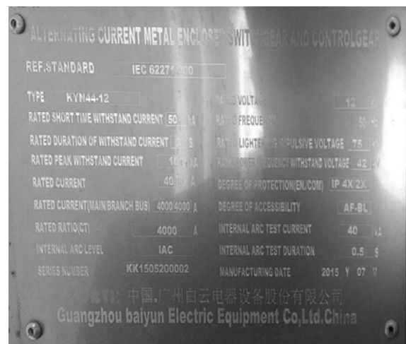
52G Breaker Nameplate
