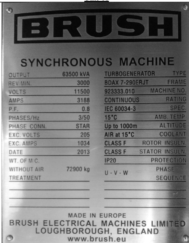
Generator Nameplate [At Actual]
