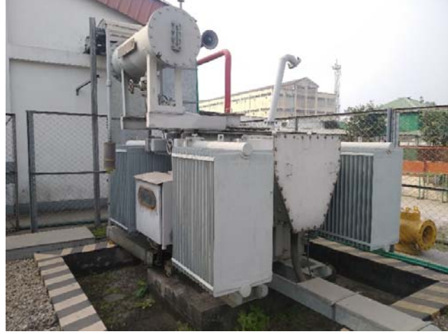
Auxiliary Transformer
