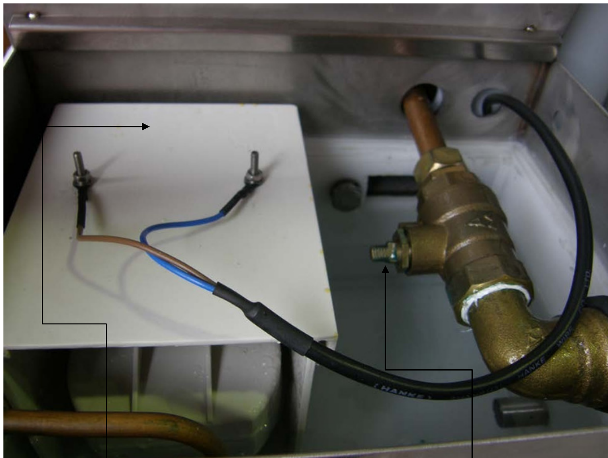
Ball float adjustment under
