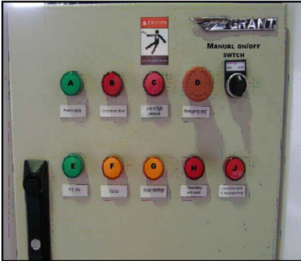
Control Panel on B400 Bin with Manual On/Off switch fitted located on Bin.
