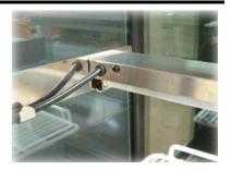
2. Lift the light assembly panel up off both shelf end supports and remove from the cabinet. The power supply cable will remain attached.
