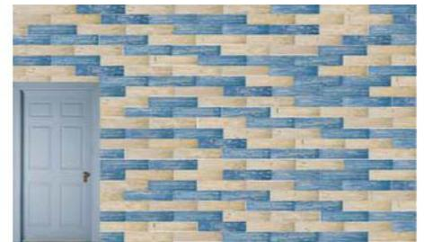
Add panels continuously until the wall is complete. Make sure the ends of the panels are aligned and that end joints are staggered. Cut the panels to size as needed.
