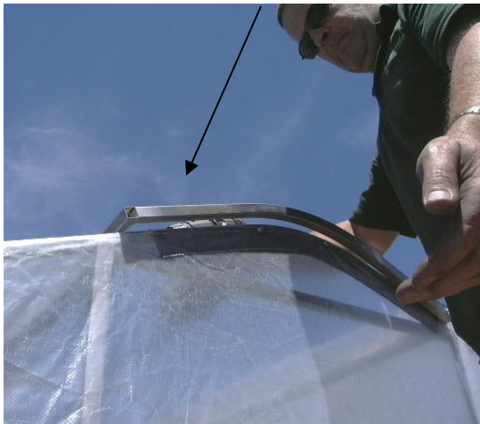
12. Re install the opening roof arches
