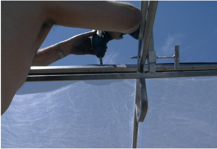
12. Re install the opening roof arches
