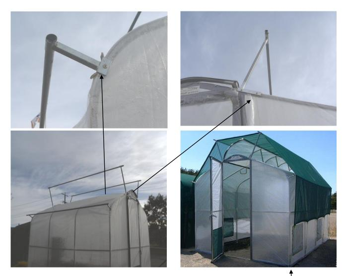
Kit comprises: Cover, Stand off brackets, self drilling screws, galvanized round pipes, bungee straps, stainless steel hooks and cable ties.
