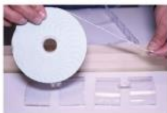
1) Cut the tape to the same length of the rail.
