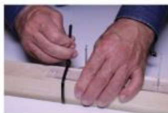
1) Wrap the flex seal tie around the rail and secure it tightly.
