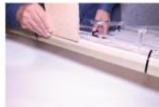
During the time of installation the modular base must be aligned, with the edge of the wall.
