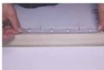
4) To finish installing, simply click the parts onto the vertical holders.
