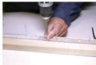
Use the holes in the rail to align the screws.
