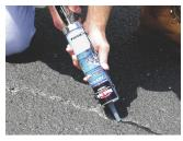
a. Fill cracks up to ½" wide with Elastic Crack Filler.
