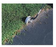
a. Trim grass and bushes away from driveway. Sweep entire surface, removing grass cuttings and other debris. Scrape clean all cracks using a screwdriver.
