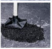
d. For holes larger & deeper than 1", use RePave Pot Hole Patch. Use tamper to pack material tight into repair. Ready for traffic immediately. Allow to cure a minimum of thirty days prior to seal coating.
