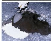
c. Repair large cracks, deteriorated surfaces, and small holes up to 1" deep with Drive-Patch. Apply with trowel, tapering into existing surface.
