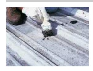
Corrugated roofing sheets are often nailed into place leaving a path for water to leak through.
