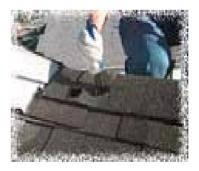
When completing a cap of shingles, the last cap will have exposed nail heads which need to be covered with Cold Process & Lap Cement.
