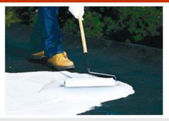
STEP 2: APPLY ELASTOMERIC COATING
