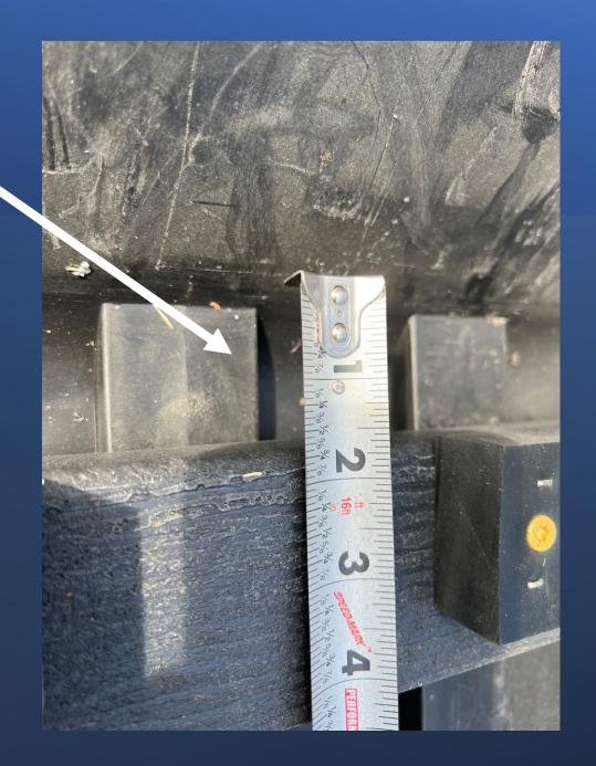
1 ½" gap provides the necessary room for the jack foot plates and the wood wedge.
