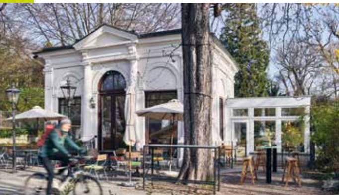
The café / gastropub Salættl is housed in a former flower pavilion that originally dates back to 1888.
