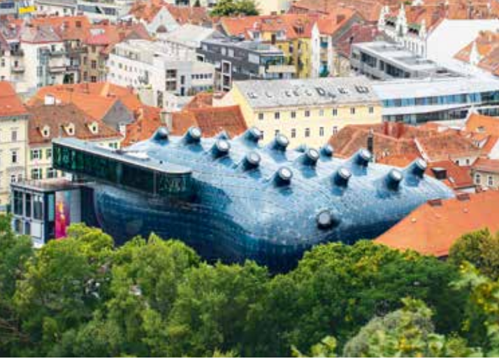
Most certainly not a white cube: the Kunsthaus, built in 2003, contributed to the city's reputation as a stronghold of architecture.
