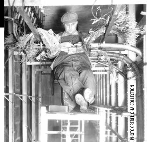
Telephone repairman splicing lines.
