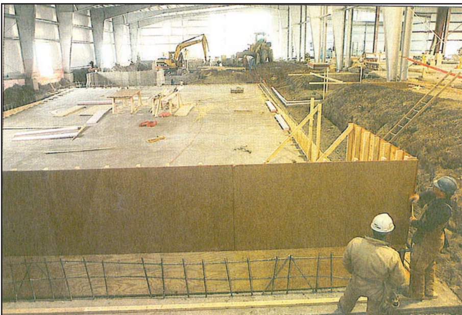
Construction on the East YMCA.
