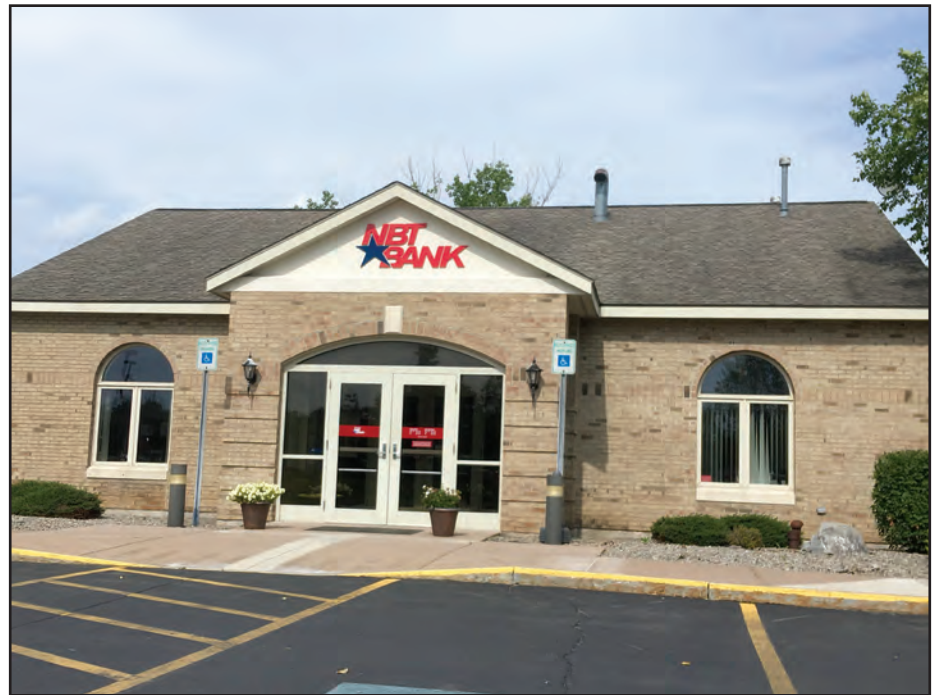
The NBT Bank branch office on Route 31 in the town of Lysander.
