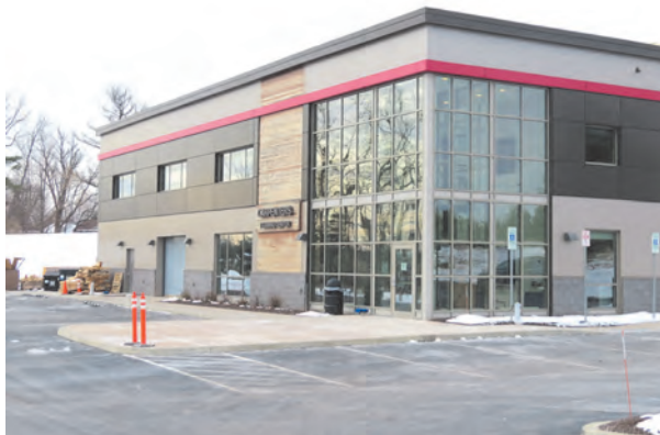
The North Atlantic States Regional Council of Carpenters (NASRCC) Syracuse Training Center is located at 6920 Princeton Ct. in the town of Salina. ERIC REINHARDT / CNYBJ
