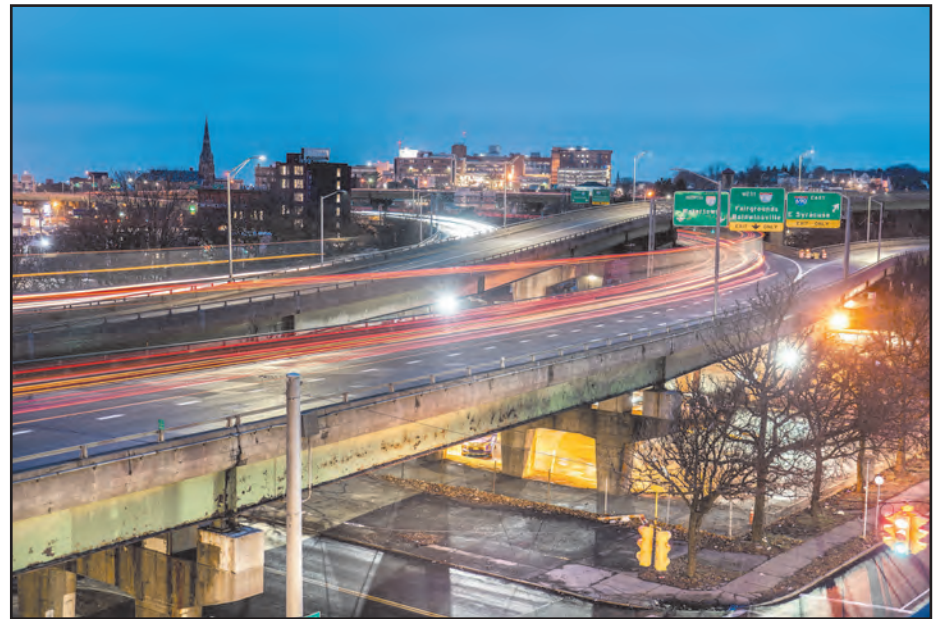
The federal government has awarded the New York State Department of Transportation and the City of Syracuse more than $180 million in funding for work on neighborhoods impacted by the Interstate 81 (I-81) viaduct-replacement project. The work will focus on streets, parks, greenery, and other community infrastructure after the elevated portion of I-81 comes down later in the decade, the office of U.S. Senate Majority Leader Charles Schumer (D-N.Y.) announced March 11.
