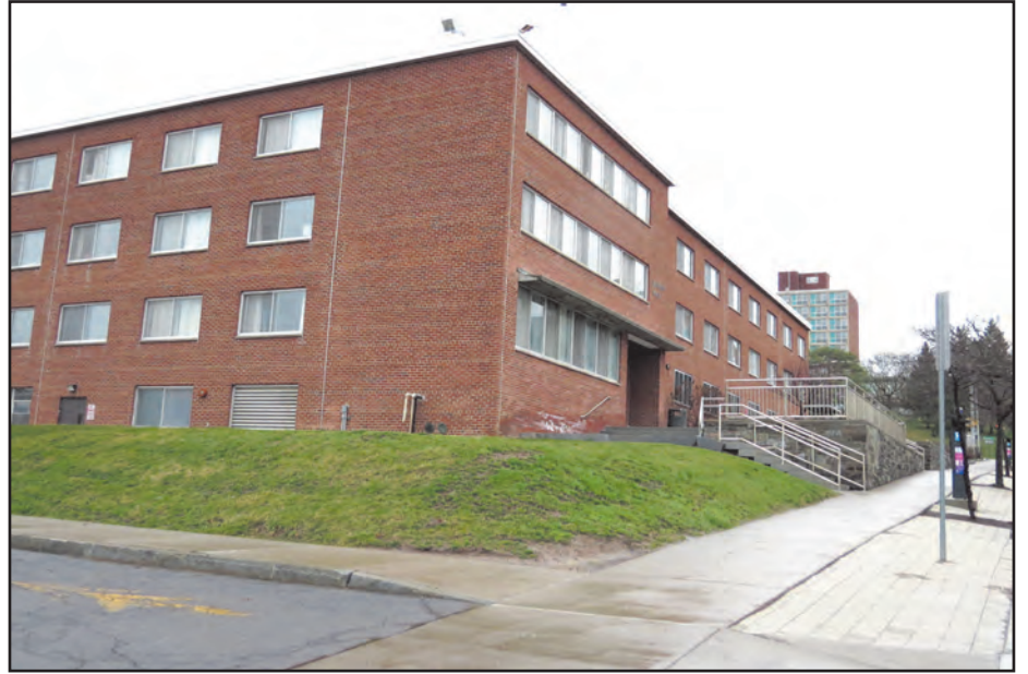
Syracuse University plans to demolish Marion Hall (pictured here on March 10) and the adjacent Kimmel Hall and dining center as part of its new housing strategy. The university will build a “modern, new” residence hall following demolition of those two buildings. Syracuse's new housing strategy, announced on Feb. 26, also includes building a new residence hall at 700 Ostrom Ave.
