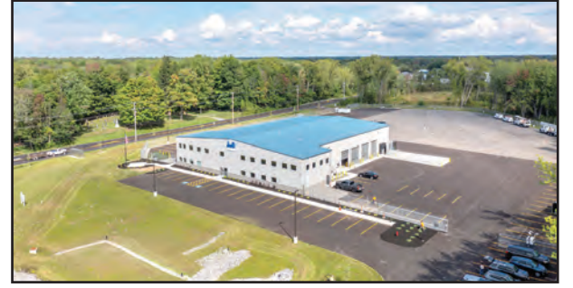
VIP Structures, a design-build firm based in Syracuse, was recently honored for its work on the J.W. Didado Electric New York headquarters building in Clay. PHOTO CREDIT: VIP STRUCTURES
