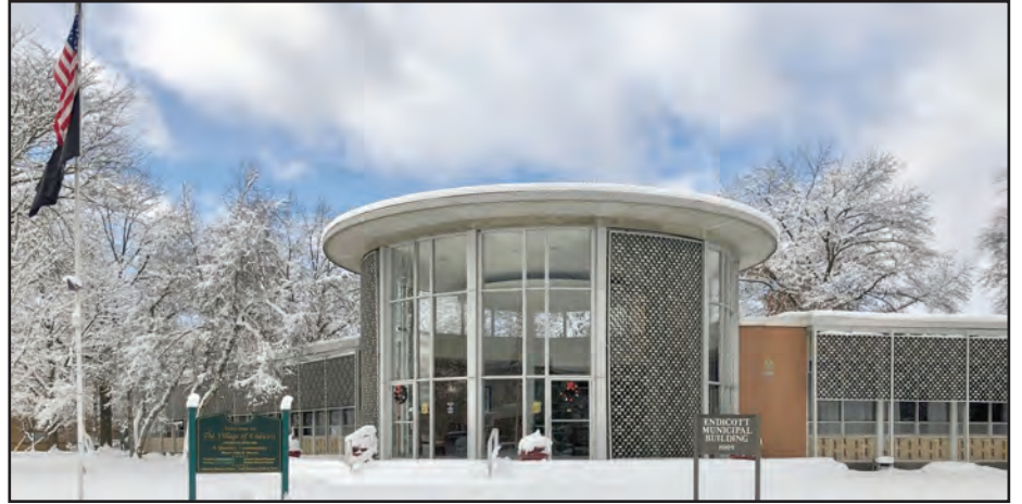
The Village of Endicott has recently received a $1.78 million state grant to make water-quality improvements. PHOTO CREDIT: VILLAGE OF ENDICOTT WEBSITE
