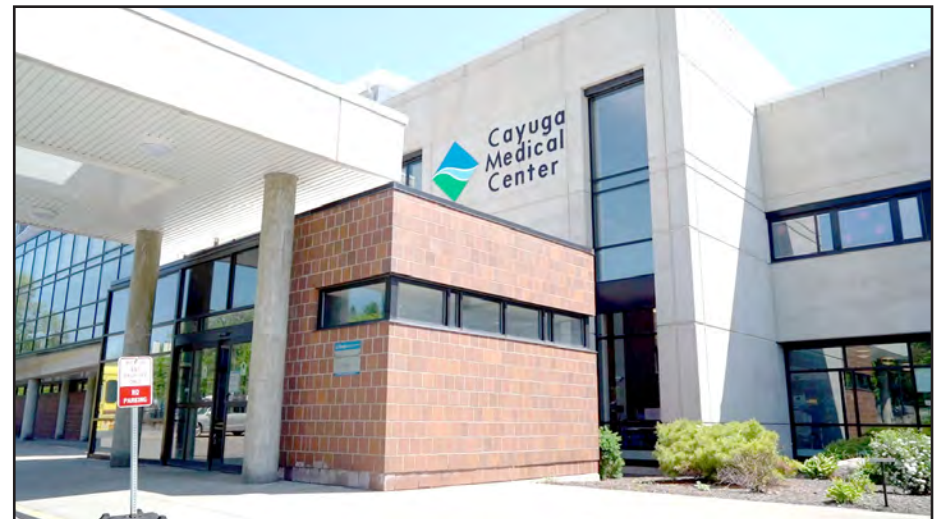
The federal government has awarded Cayuga Medical Center in Ithaca more than $10 million to reimburse the cost of installing two generators, an underground storage tank, a new building to house the generators to keep the hospital operational during extreme-weather events. PHOTO CREDIT: CAYUGA HEALTH
