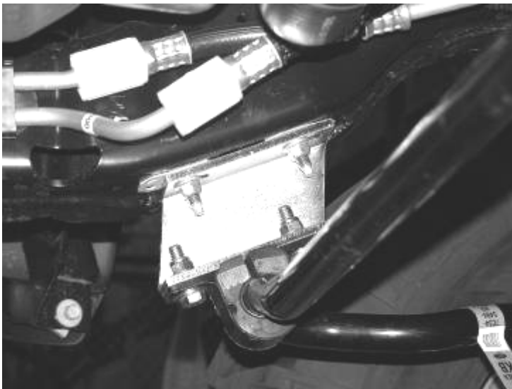
View of inner passenger side frame rail
