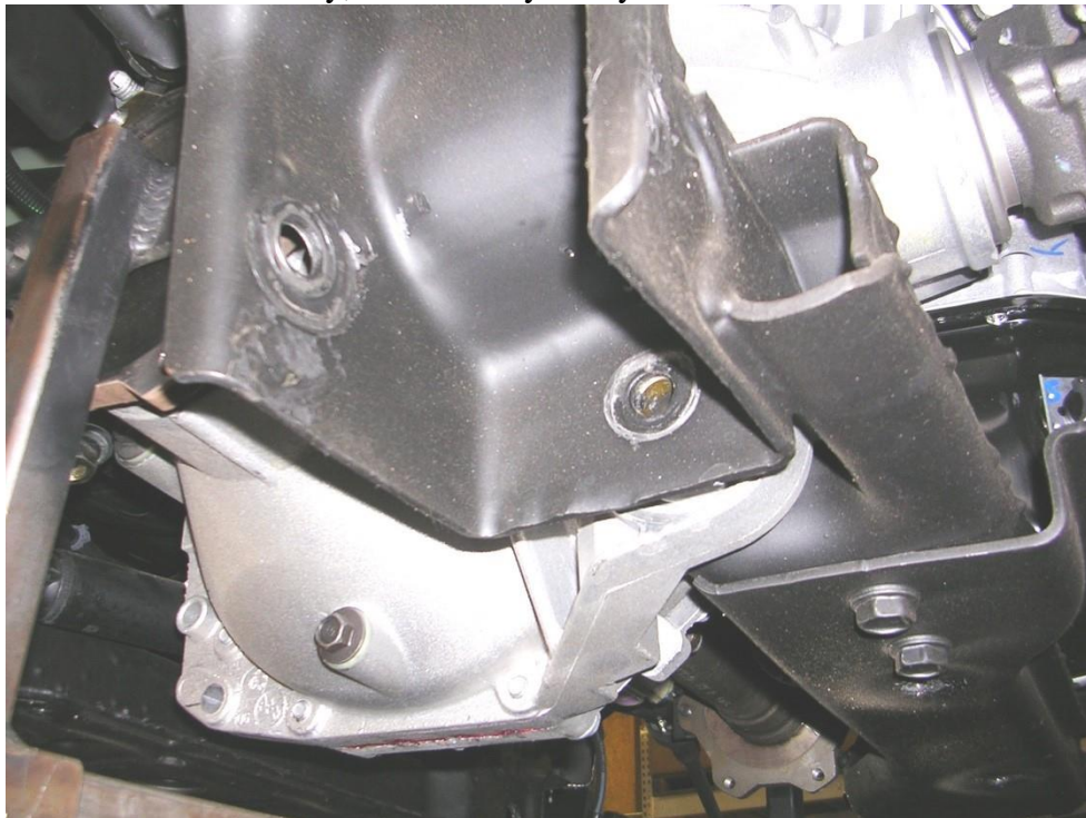
Figure 11: Lower bolt removed from front differential prior to making frame cut.
