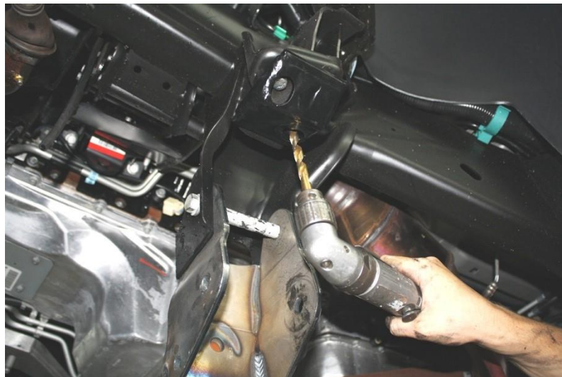
Figure 12: drill mounting hole for bump stop brackets
