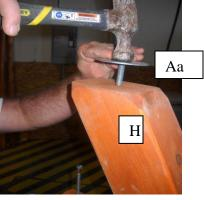
**Step 9:** Use a 20" brace (**J**) on each side of the table legs (**H**) to and attach it to the seat bottom braces (**B**) (as shown). Use 2 ½" lag bolts (**I**) through pre-drilled holes in all 8 braces (**J**). Use ½" washer (**W**) when fastening lag bolt. Place t-nut (**Bb**) with prongs facing down and tap into pre-drilled hole on end of table leg. Screw leveler (**Aa**) into t-nut (**Bb**). Place table upright and adjust metal leveling screws (**Aa**) as needed.
