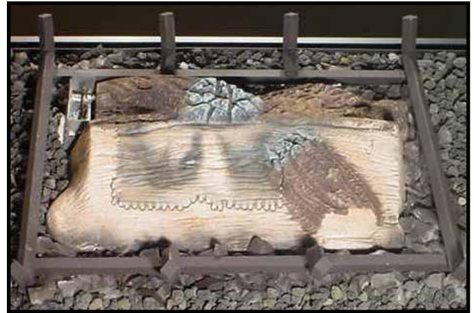
Figure 9.5 Placement of Lava Rock
