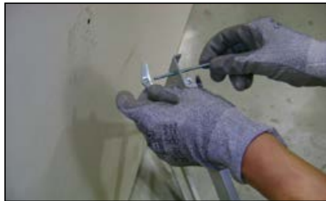
Figure 4.5 Toggle Bolt Installation through Mounting Bracket
