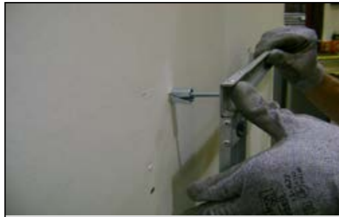
Figure 4.6 Installing Anchors in Hollow Wall
