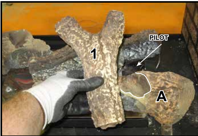
Figure 3. Placement of Log #1
