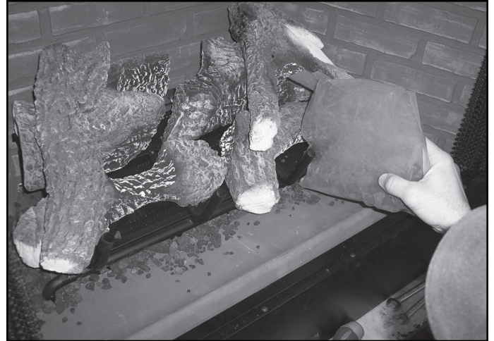
Figure 14.21 Placement of Lava Rock
