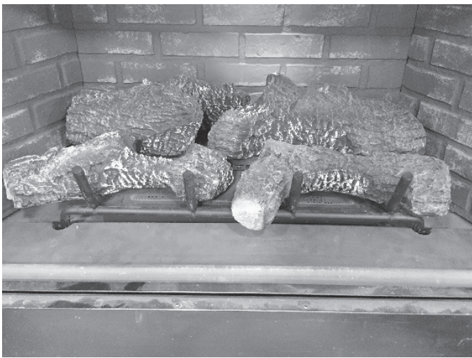
Figure 14.13 Left and Right Front Log Placement
