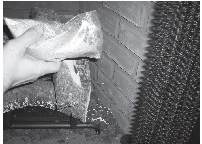
Figure 14.22 Placement of Vermiculite
