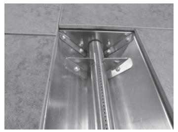
Figure 5.4 Pan Installed Under Finish Material
