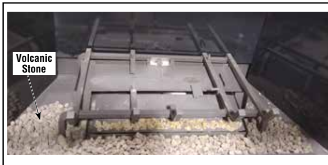
Figure 40 - Install volcanic stone
