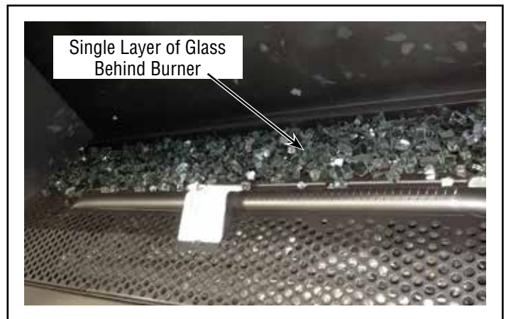
Figure 45B - Placing a Single Layer of Glass Media.
