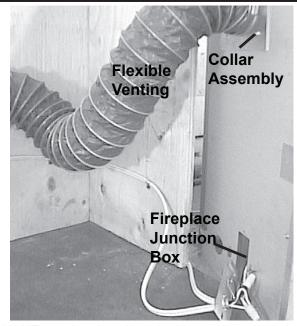
**Model NZ26:** when installing the kit on this model, the collar assembly must be secured to the duct cover plate located on the base of the unit only.
