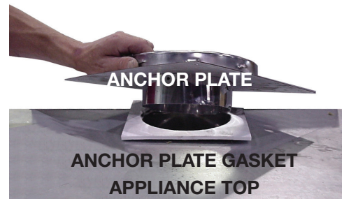
ANCHOR PLATE FOR A FACTORY BUILT CHIMNEY
